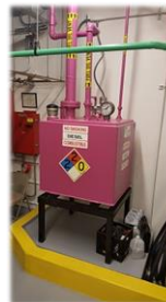
Top left – day tank for an emergency generator
